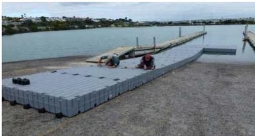
Above - The pontoons being assembled on the boat ramp & floated into the water as the structure took shape
