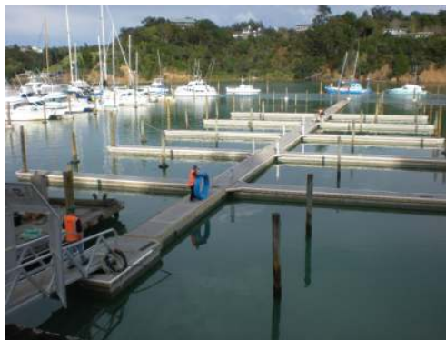
The almost finished D Pier
